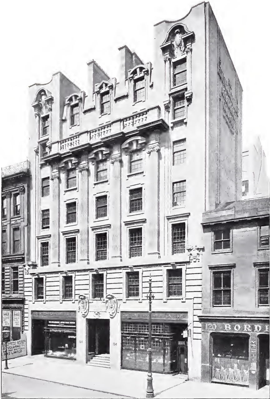
776. Edinburgh Life Assurance Company , JOHN A. CAMPBELL, Architect. Mason: Morrison and Mason, Polmadie, Glasgow. Fireproof Flooring: D. Ferguson and Co., Glasgow.
